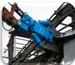
Crushers for demolition of buildings (steel frame cutters)
