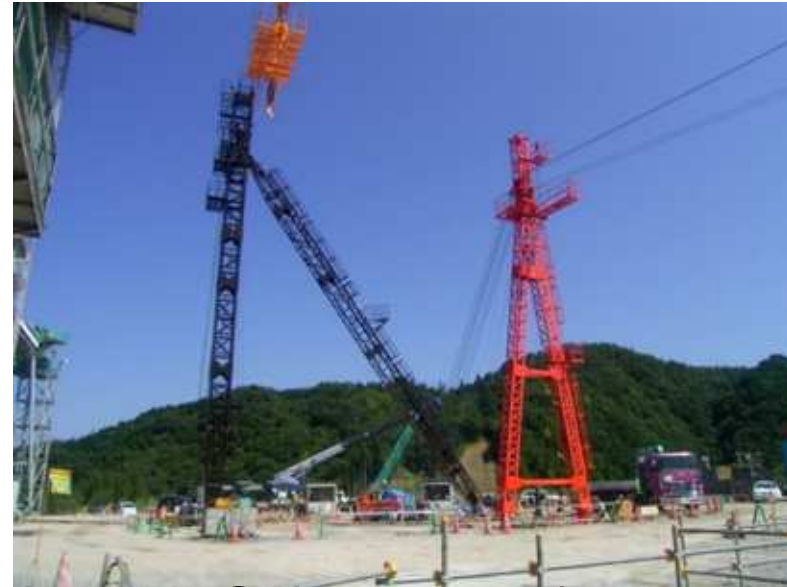
Cable crane for dam construction
