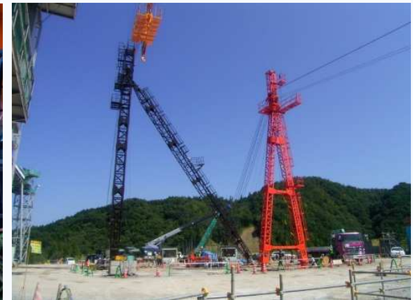
Cable crane for dam construction 3
